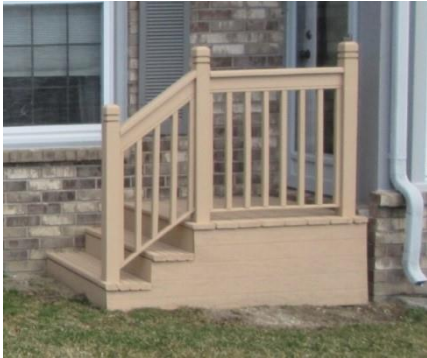
Platform steps and railing in pressure treated lumber for Brookfield great room .
